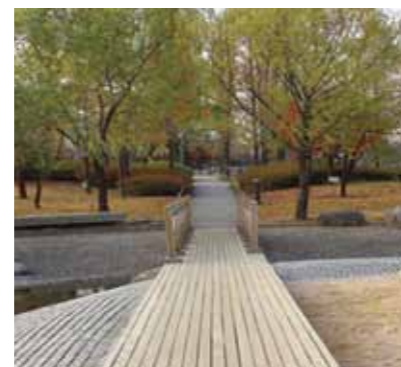
Pedestrian bridge over the Nallah
