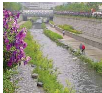
Pedestrian bridge over the Nallah
