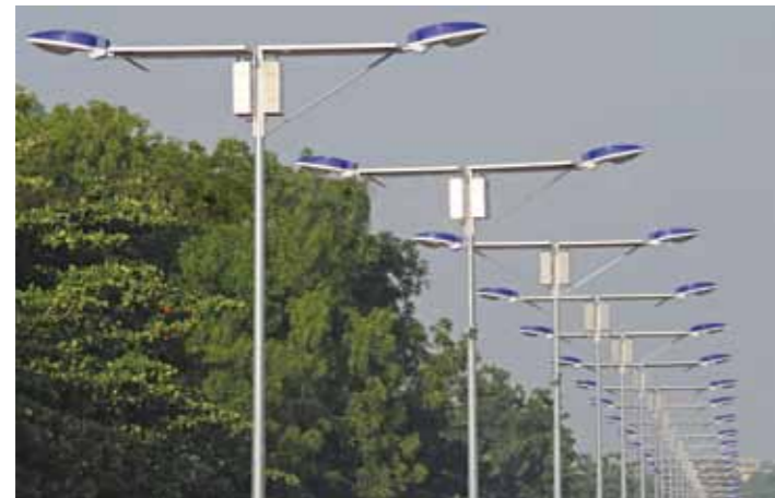
Solar Street Lights
