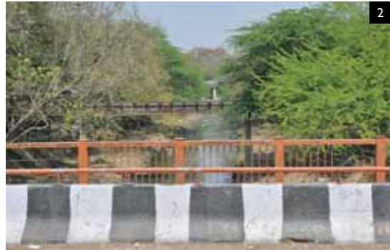
Satpula Drain viewed from the roadside
