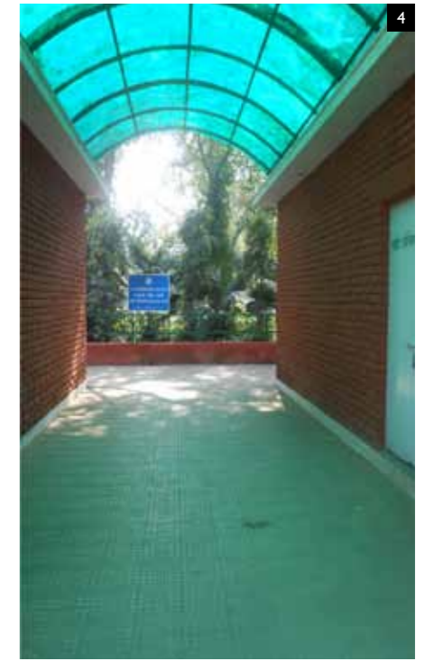
Existing DDA site office
