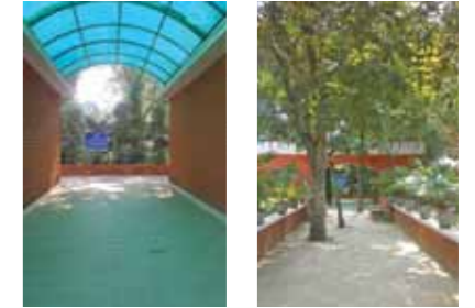
Node 3: Existing DDA Site Office
